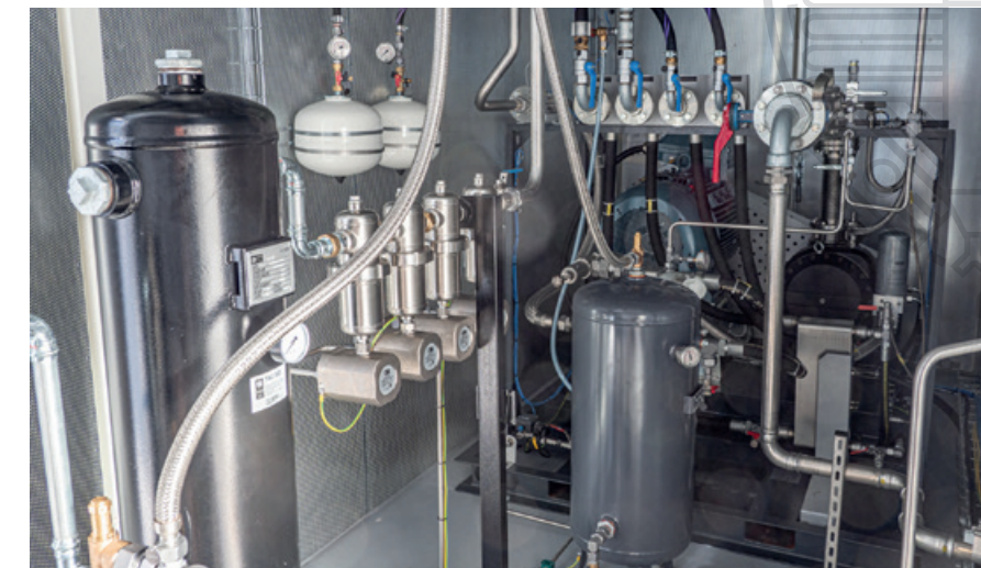
Water-cooled CNK9-55 screw compressor
